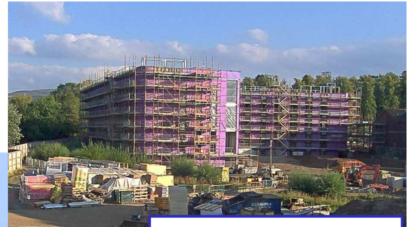
Under construction.. Charles Lyell Centre Heriot-Watt University
