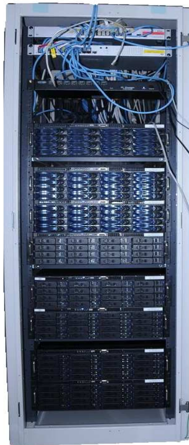
Figure 3. The K5/VSI system installed in the Mitaka correlator room
