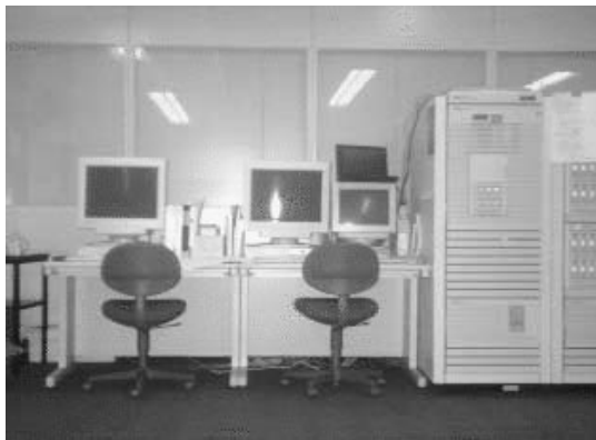
Figure 1. System control workstation and its terminals.
