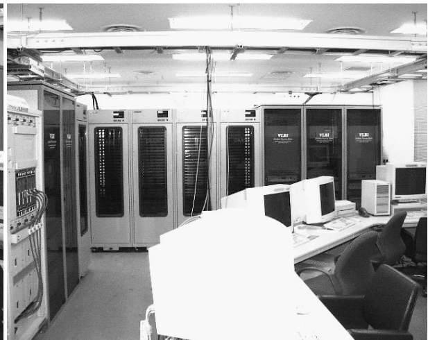
Figure 7. View of the correlation processing system.
