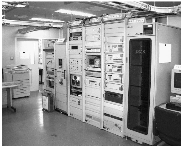
Figure 6. View of the data-acquisition system.
