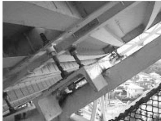
*Figure 3. Corroded nut plate which fasten the main reflector to the back structure.*
