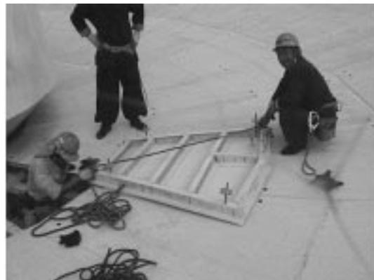
*Figure 4. Removing main reflector panel for replacing the nut plate.*
