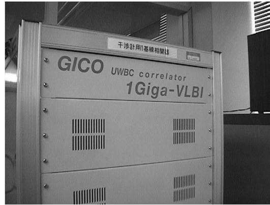
Figure 1. Newly installed front panel of the UWBC-GICO correlator.
