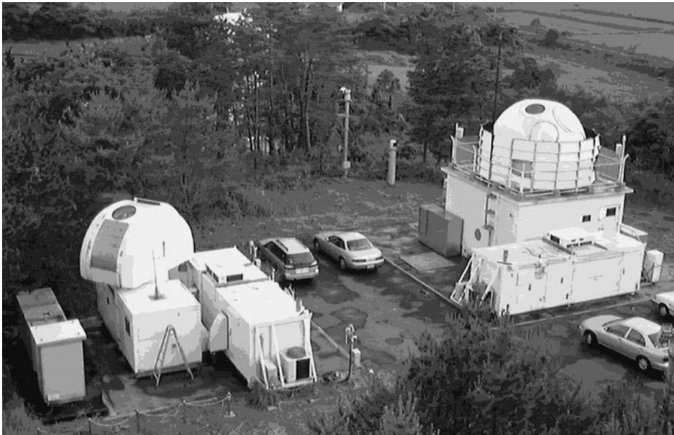
Figure 1. The Kashima station and the mobile station used to detect the reflected pulses. The baseline vector in the direction of the mobile station from the Kashima station lies in the west-east direction and is about 20 m in length.
