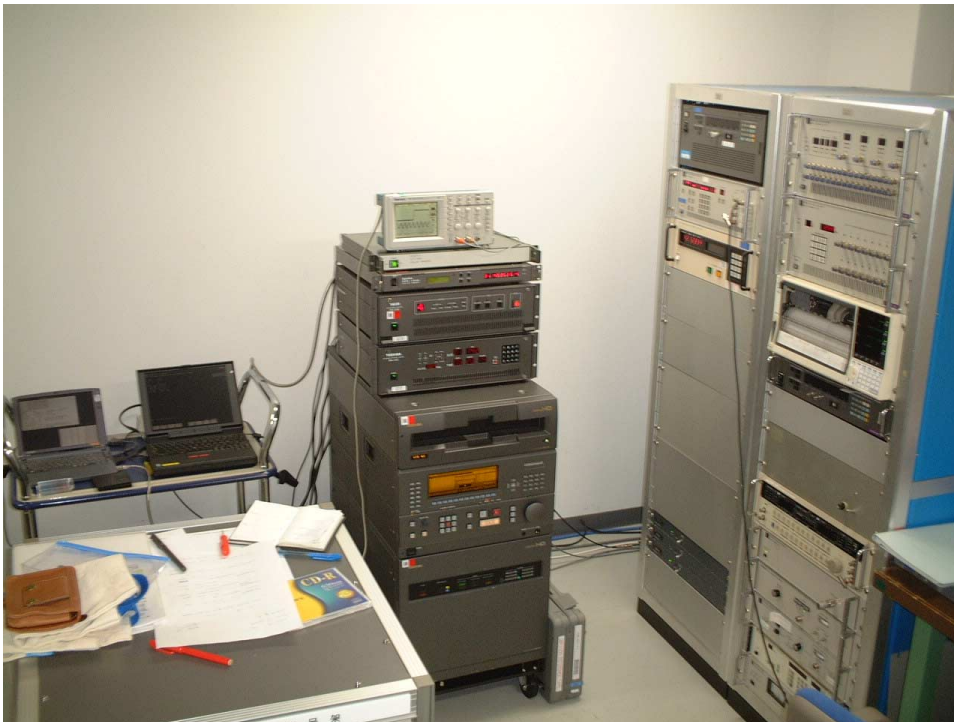
Figure 2. The Gbit recorder installed at the Mizusawa station temporarily. Currently two portable PC are used to control. One is for the observation and another is for the ftp-VLBI. These PC-based field system will be unified.
