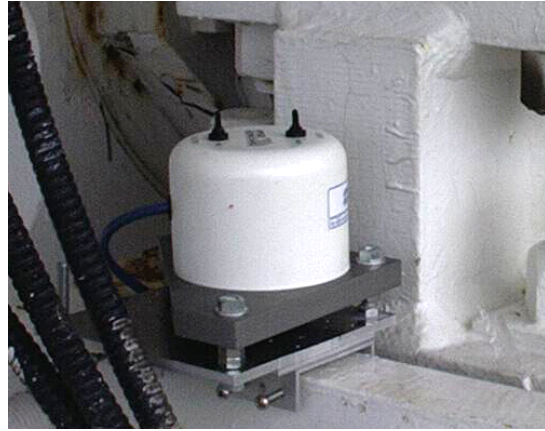
Figure 1. Inclinometer embedded on antenna structure.
