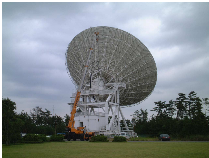
Photo. 34m telescope and a crane truck. Elevation motors are removed and sent back to the factory for overhaul. (see topics on page 4 for details)
