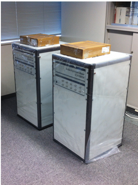
Figure 3. Hydrogen masers and remote monitoring and controlling system.
