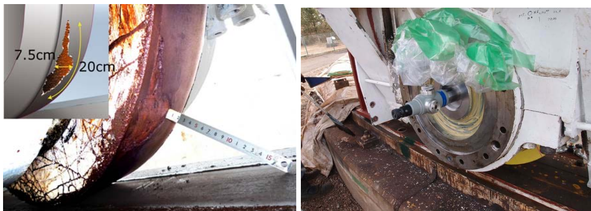
Figure 1. Left panel shows the crack on the wheel with 20cm/7.5cm size. Right panel indicates the installation of new wheel, whose axis is accurately aligned to the center of the azimuthal axis by using a telescope.
