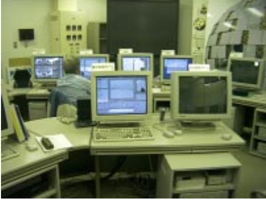
(a) control center
