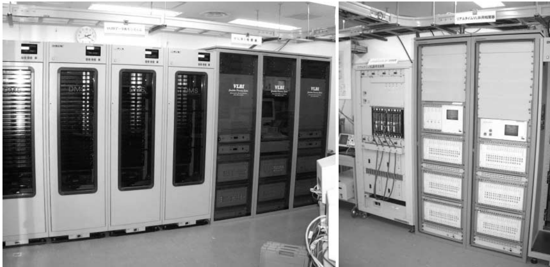
Figure 1. The KSP tape-based VLBI correlation system (left) and the KSP real-time VLBI correlation system (right) at Koganei. In the left figure, four racks at the left are automatic tape changer (DMS-24). The right three racks contains correlators, output interfaces, and correlation controller. All of these tape-based equipment will be transported to Kashima Space Research Center in near future.
