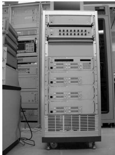
Figure 5. Prototype K5 system. From top to bottom, a reference signal distributor, 16-ch video amplifiers with low-pass filters, and 4 PCs for VSSP boards.
