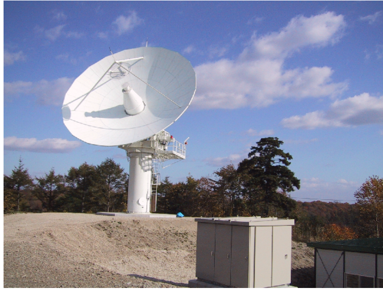
Figure 2. 11-m VLBI antenna at Tomakomai Experimental Forest of the Hokkaido University. The antenna and the VLBI observation facilities were transported from Miura KSP VLBI station in early 2001.
