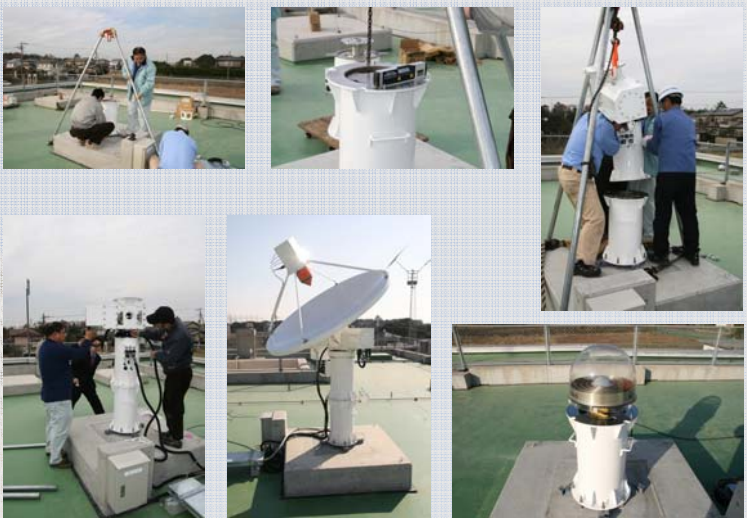
Figure 5 Installation of a first prototype of the compact VLBI system on the top of the 34 m antenna building on December 9, 2008 at Kashima.
