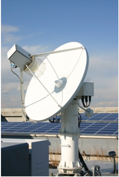
1.5 meter antenna on the roof
