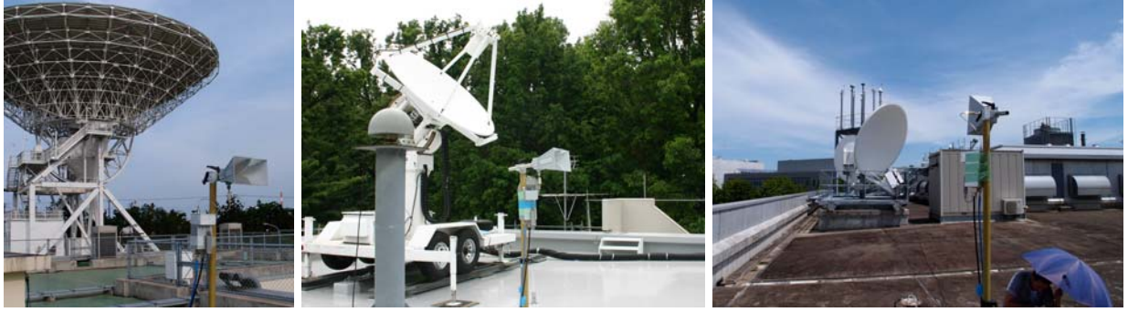
Figure 8: Picture of the measurement locations: (A) Left: At the roof of Kashima-34m-antenna operation building. (B) Center: At the roof of operation building of Koganei 11m station, (C)Right: At the roof of National Metrology Institute of Japan(NMIJ) building.
