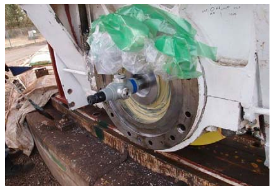
Fig. 2 Installation work of new azimuth wheel.
