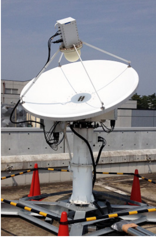
Figure 3. MARBLE1 station installed at the top of 3-7 building of NMIJ at Tsukuba.
