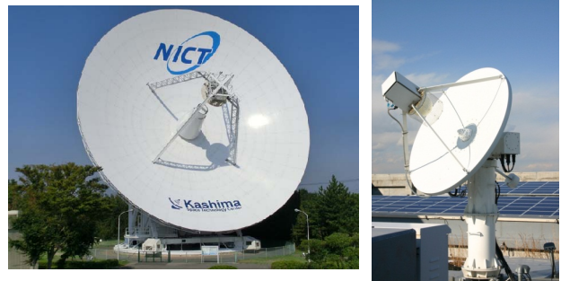
Figure 1, Kashima 34m antenna (Left) and 1.5-m parabolic antenna (right) are the components of the Gala-V system.
