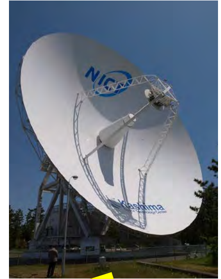
34 meter RT in Kashima
