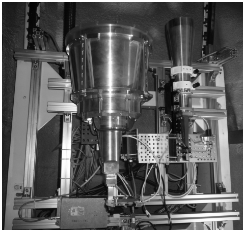
Fig. 2 Broadband NINJA feed has been installed in the receiver room of the Kashima 34-m telescope.
