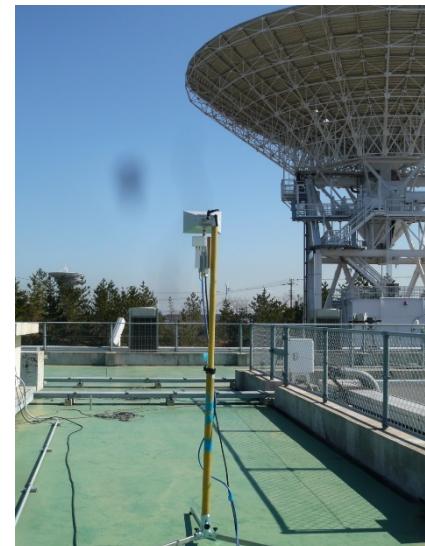
Roof Floor of Kashima 34m VLBI station Building.
