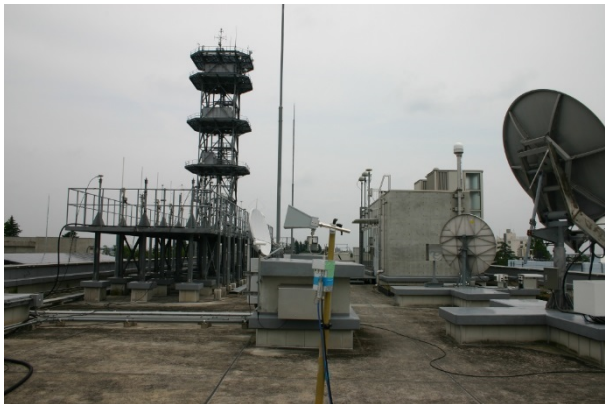
RF of 2 nd Building. Communication Antenna for TWSFTT(14GHz), Other emission from experimental system of NICT Labs.
