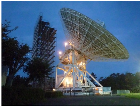
Fig. 6 Kashima 34-m antenna in holographic observation after reflector adjustment. We carried out reflector adjustment in day time and holography observation in the evening. We repeated this procedure for a week. For safety, we have watched the antenna during the holography observation about 1.5 hours to avoid accidental smash with the scaffolding.
