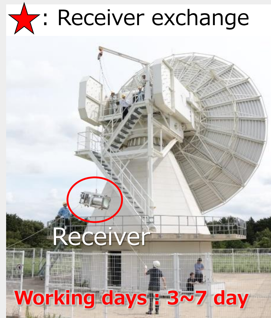
Figure 1. Observation schedule for the Ishioka Station in a certain year (left). Working scene of receiver exchange at the Ishioka Station (right).
