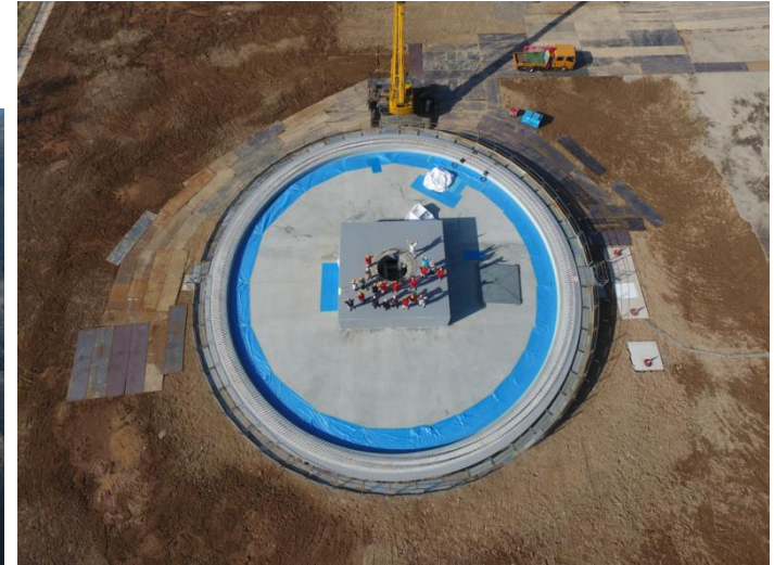
↑ Antenna Foundation (No Az rail)
