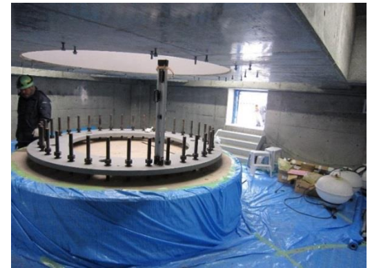
Foundation of Master Collimator
