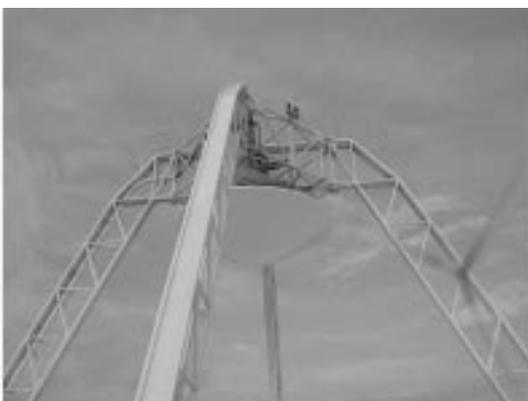
*Figure 2. Placement of the subreflector in a normal position.*
