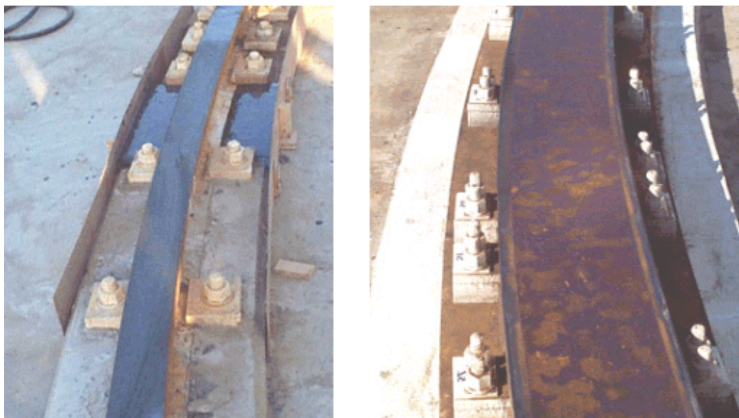
Figure 2. The replaced rail (Left: before, Right: current).
