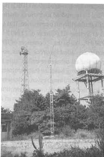
Fig. 2 A crossed 3-element Yagi antenna system at Kashima (Kashima-B).
