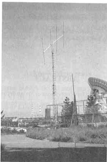
Fig. 1 A crossed 4-element Yagi antenna system at Kashima (Kashima-A).
